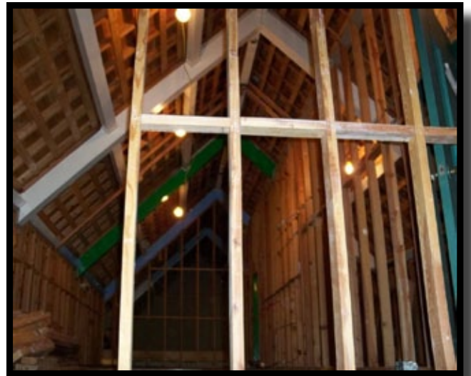
Upstairs Willcox building interior
